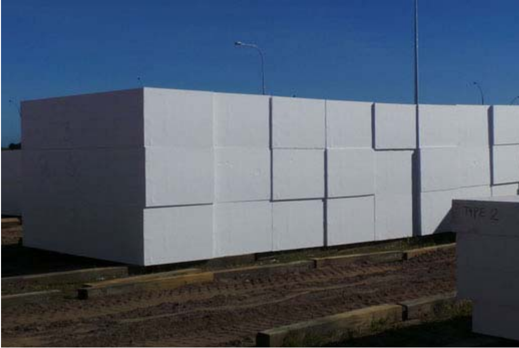
Polystyrene blocks at the TEL construction site.
