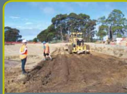
1 Fill is laid to construct the first MSE wall layer.
