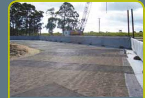
3 Geo-grid mesh and fabric is laid.
