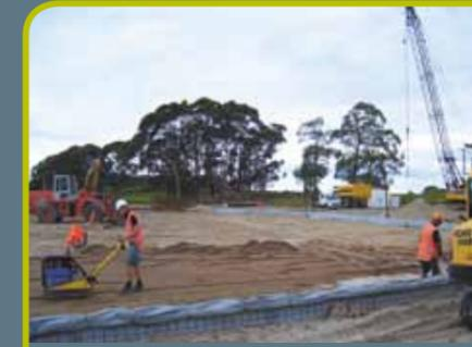
2 Fill material compacted in preparation for the next layer.
