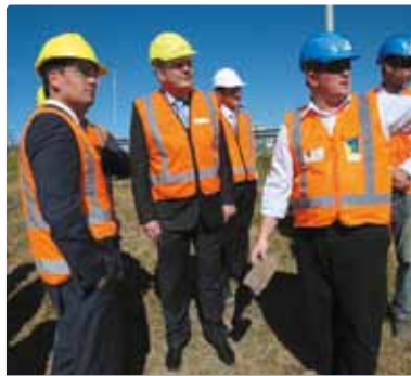
Fulton Hogan HEB Construction Alliance project director Andrew McRae explains the Domain Road ground improvements (wick drains).
